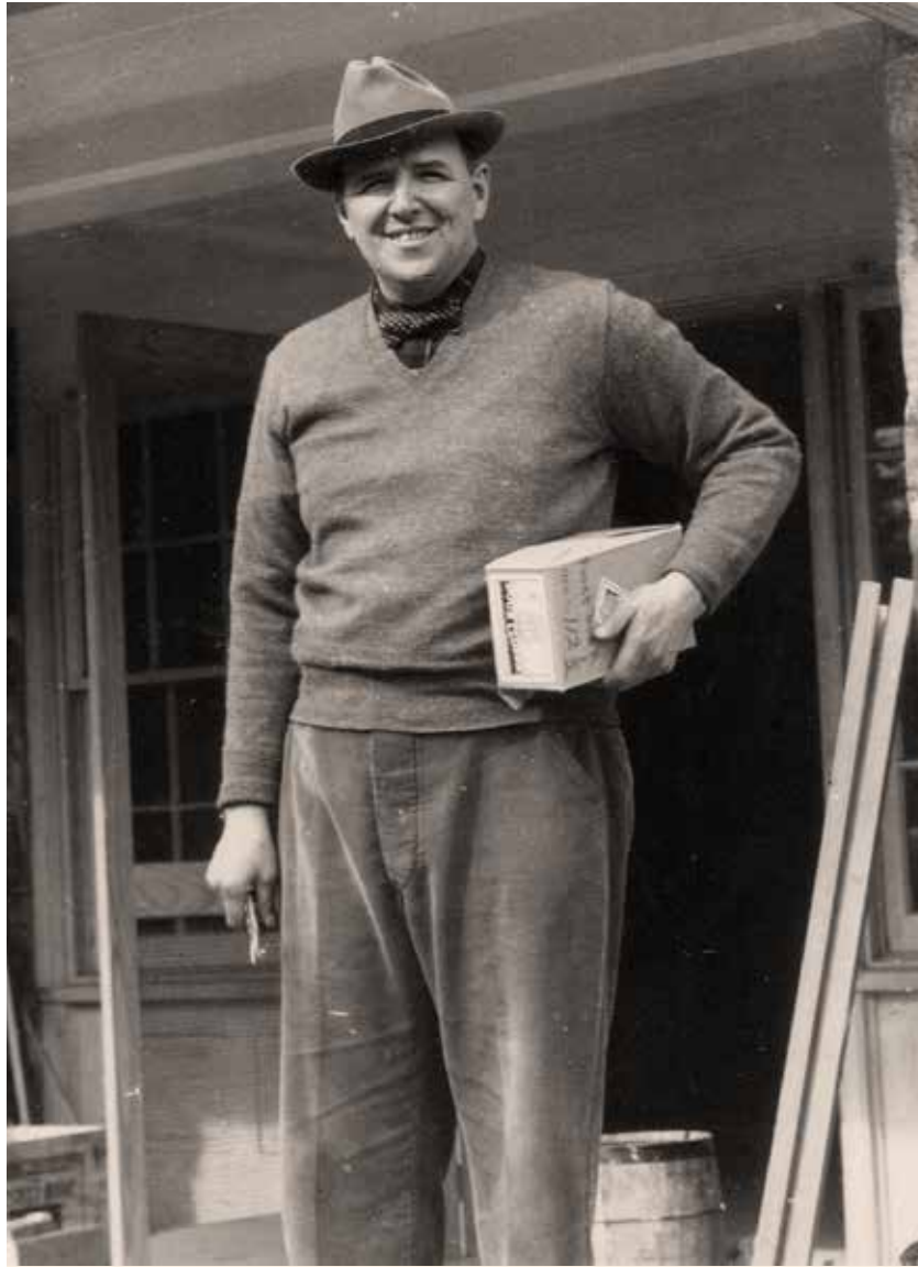
Dave Lasier on the work site in 1941.
